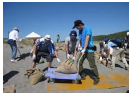
Piling up sandbags
