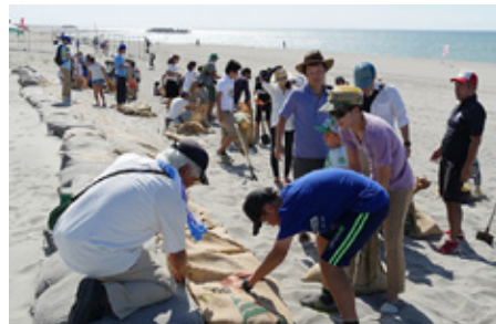
Sand-filled cloth bags prevent sand from washing and blowing away
