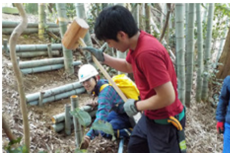
Building bamboo stairs
