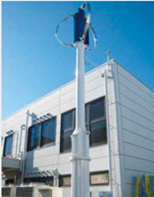
Vertical wind power generation system, which is quieter than the propeller type (Nakaze Factory)
